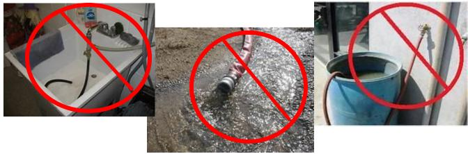
When the water supply system experiences increased or decreased pressure (such as when the lines are being flushed, a repair is being made, or there is a break in the water line), **<u>backflow</u>** from the non-potable source can contaminate the potable water source.
